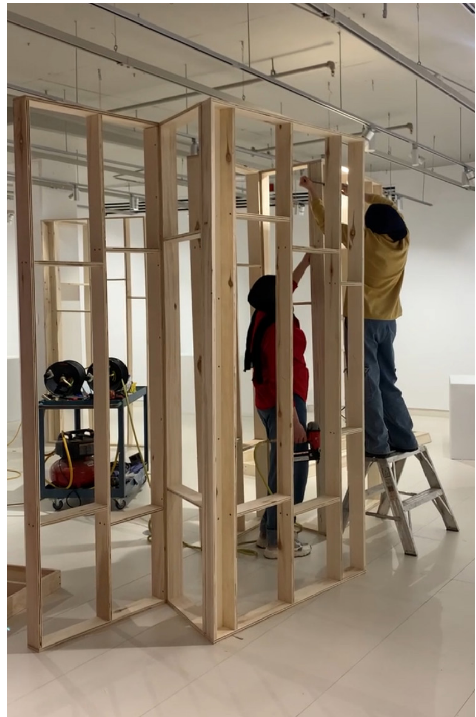
Construction of wall
